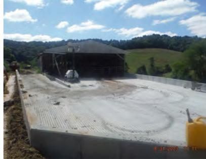
**Cree Before 2:** This photo shows the two lots that have been concreted and reinforced with retaining walls. The new concrete heavy uses area will significantly reduce the nutrient runoff to the stream located right of the lot.]
